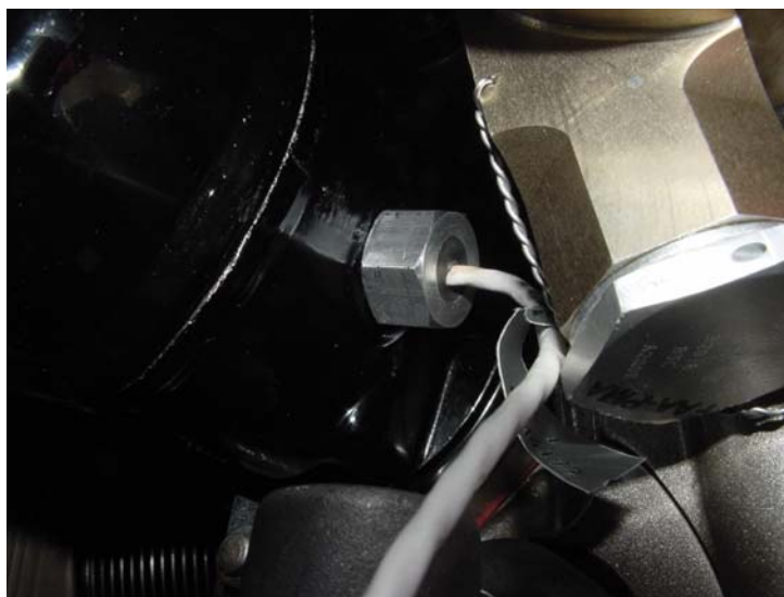
Figure 5-13. Magnetic Tach Sensor Installed
