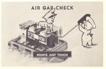
To adjust the air gap, insert gauge between armature and core, press armature down against gauge, loosen the two contact mounting screws and raise or lower the
