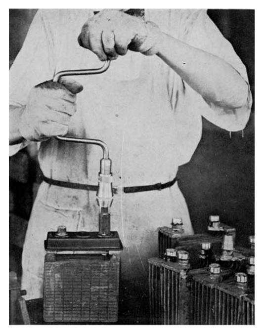
Fig. 249. Reaming Prest-O-Lite Peened Post to Remove Cover
