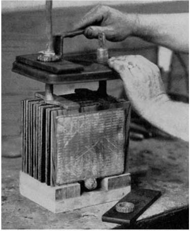
Fig. 313. Fastening Cover. Delco-Light Cell
