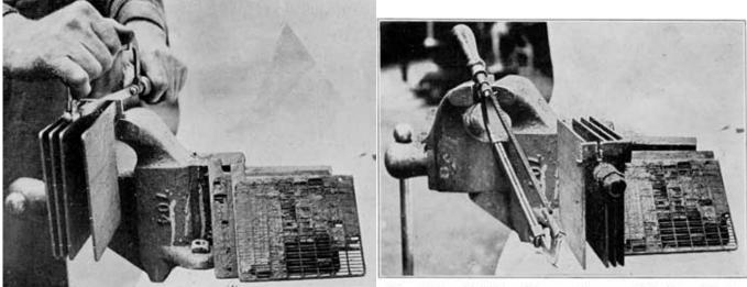
Fig. 148. Sawing Slot in Plate Strap
