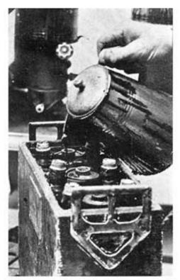
Fig. 229. Pouring Compound on Lower Covers
