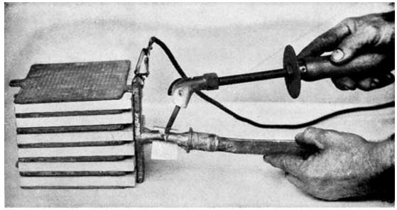
Fig. 317. Repairing Broken Post. Delco-Light Cell
