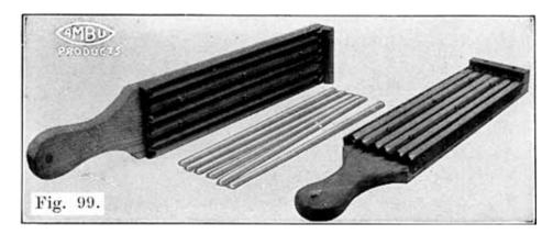
Fig. 99. Burning-Lead Moulds, and Burning Sticks Cast in Them
