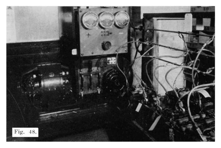
Fig. 48. Hobart Bros. Co. 3 K. W. Constant Potential Motor-Generator Charging Set
