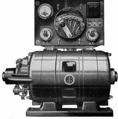
Fig. 45. Ten Battery Motor-Generator Charging Set
