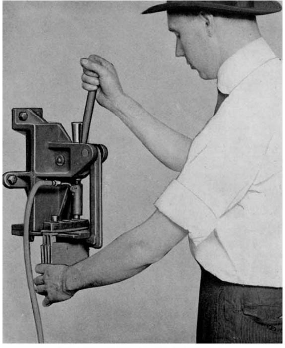
Fig. 253. Peening Prest-O-Lite Post with Special Peening Press
