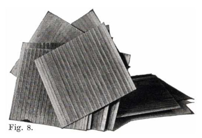
Fig. 8. A Pile of Prepared Wooden Seperators Ready to be Put Between the Positive and Negative Plates to Form the Complete Element.
