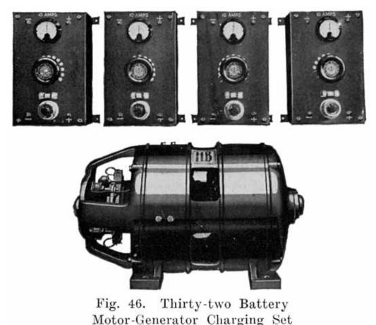
In choosing a charging outfit, it is important not to get one which is too large, as the outfit will operate at a loss when running under a minimum load. It is equally important not to get one which is too small, as it will not be able to take of the batteries fast enough, and there will be a "waiting list" of batteries which cannot be charged until others are taken
