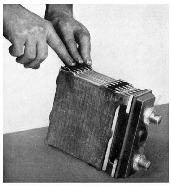
Fig. 268. Inserting Vesta Hard Rubber Isolator
