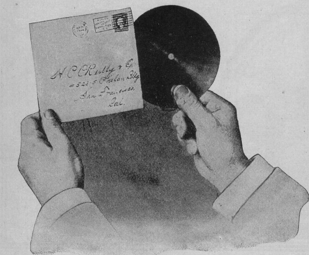
The Latest Telegraphone "Dictation" in the Form of Thin Steel Discs May be Mailed; the Recipient Transcribing the Speech Record on His Machine.
