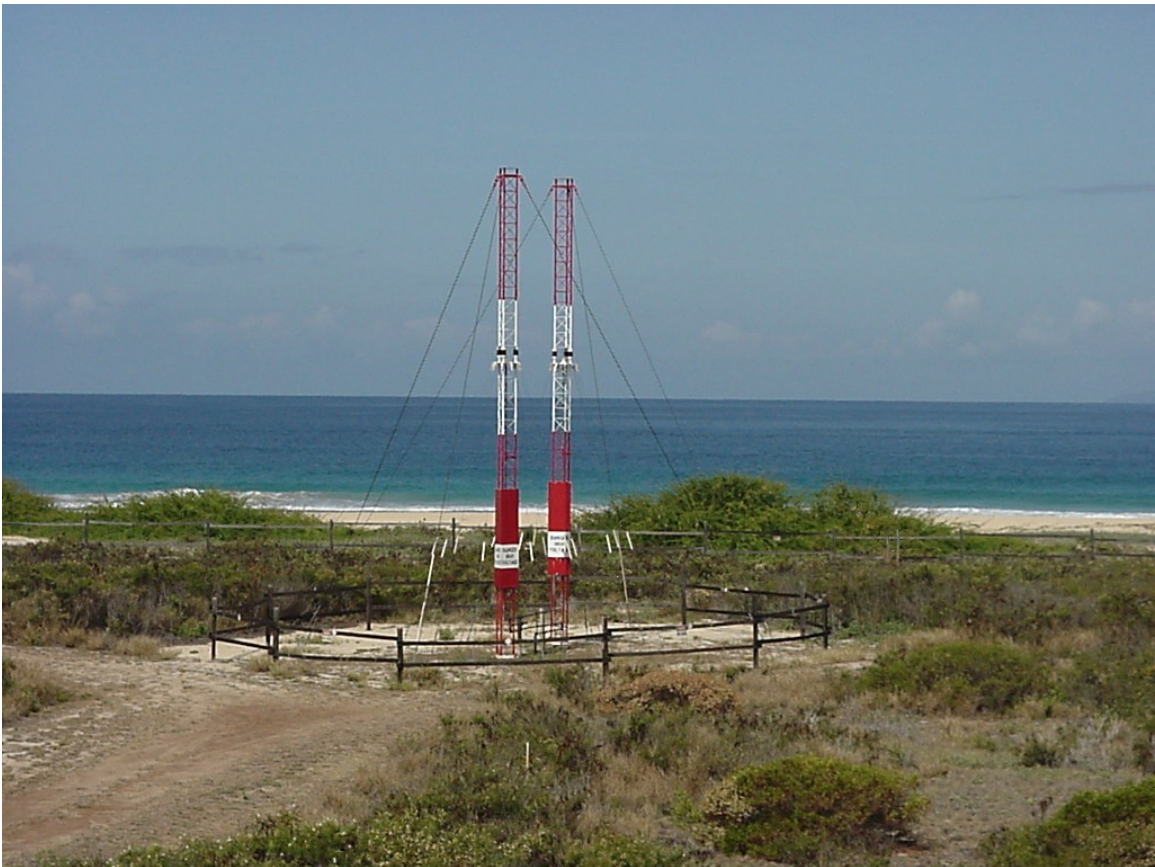
Figure 1.29. 15 MHz antenna at WWVH.
