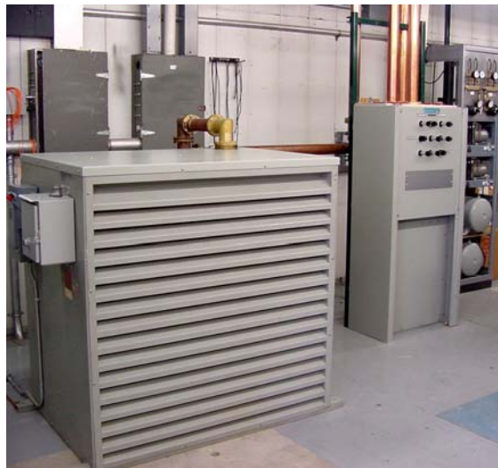
Figure 1.18. Dummy load and switch matrix..
