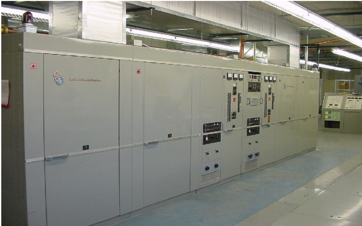
Figure 1.16. WWVB transmitter.
