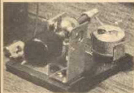
The crystal/whisker act as a rectifier diode to detect audio from the tuned LC circuit.
